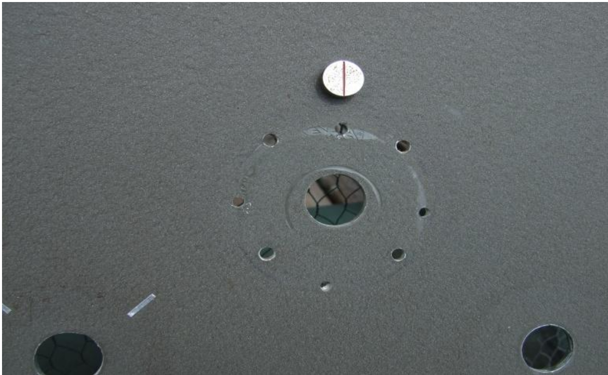
Fig. 3 Mounting holes for slow-motion drive
